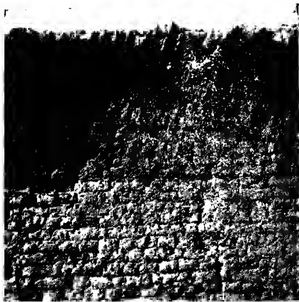
Fig. 2. — DETAIL OF COPTIC MUD-BRICK LAMINATED VAULT WITH LEANING COURSES (SAQQARA).
